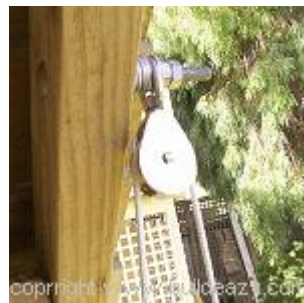
The pulley hanging loosely from a bolt through the rafter.
