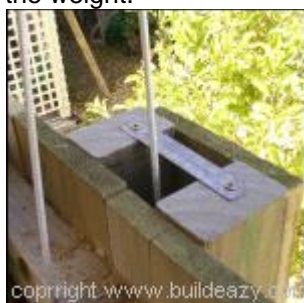
Metal strap across top of case to ensure weight cannot be pulled out. Put one on the bottom as well.
