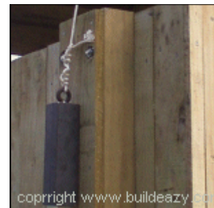
The weight before being dropped in the casing. Tie the weight well.
